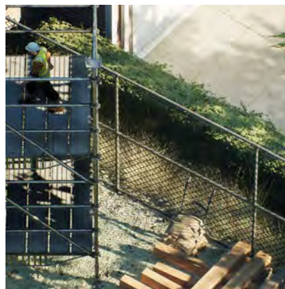
Fig.25. a lot of construction going on
