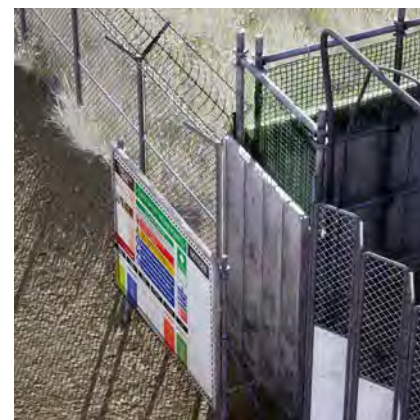
Fig.28. traditional constructions produce breaks
